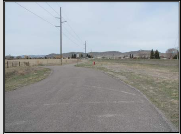
Figure 2. Existing Highway 41 Trail
