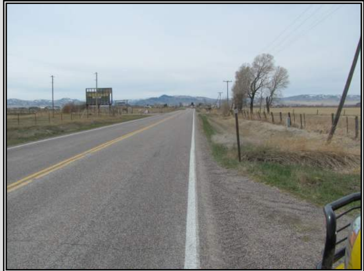
Figure 13. Highway 91 South Looking South
