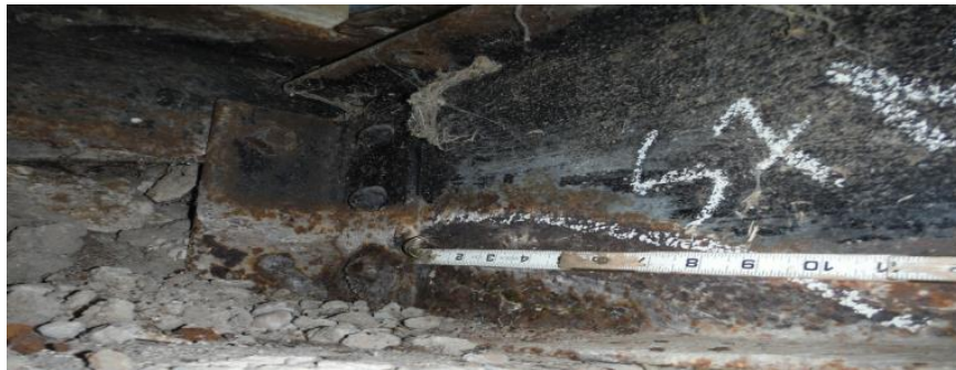
Figure 15: View of 100% section loss through web of Stringer 7 at Abutment 2 (courtesy of MDT)
