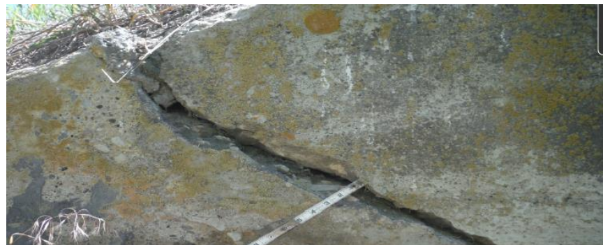
Figure 11: View of 1" wide crack in Abutment 2, north wingwall, typical of wingwall cracking (courtesy of MDT)
