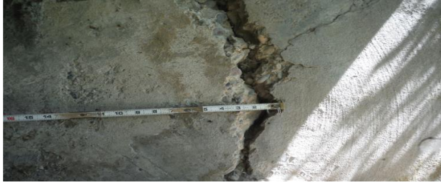
Figure 12: View of Abutment 2 full height vertical cracking up to 1 ½" wide adjacent to the south bearings (courtesy of MDT)
