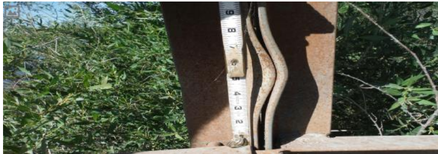
Figure 13: View of 1" distortion in north truss vertical, common in several areas throughout (courtesy of MDT)
