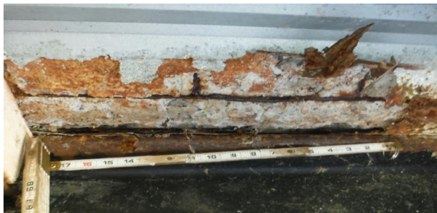
Figure 9: View of deck underside with area of exposed and corroded reinforcement. Note lack of steel stay in place form (courtesy of MDT)
