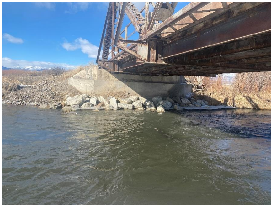
Figure 6: View of mitigated undermining area at Abutment 1 with riprap in 2022.
