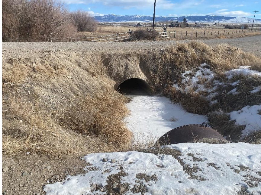
Figure 7: View of corrugated steel pipe crossing for Staudaheer – Bishop Ditch under Anderson Lane. The other pipe in the foreground is the boiler pipe crossing under the access road that is attached to the headgate. Note steepness and roadside safety hazard of the open ditch section.
