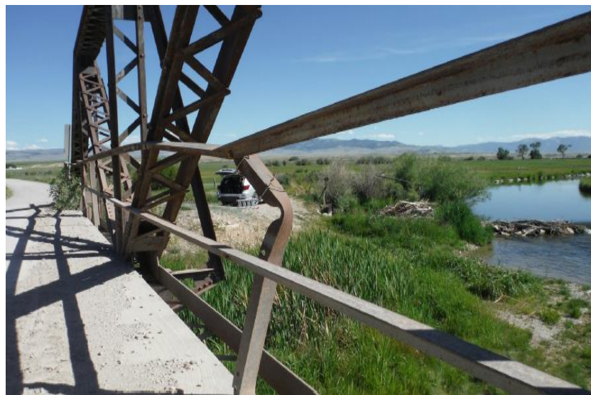
Figure 20: View of substandard original bridge rail, with area of damage (Courtest of MDT)
