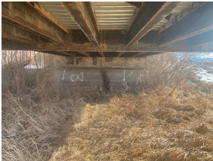
Figure 17: General view of bridge underside, note coating failures typical.
