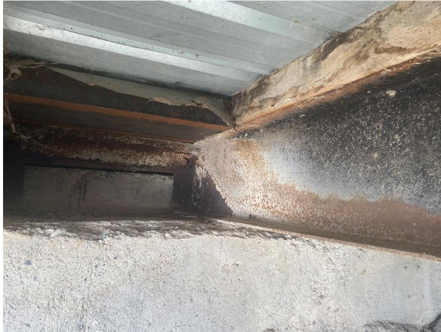
Figure 10: Typical view of spalling and abrasion over length of top surface of abutment.
