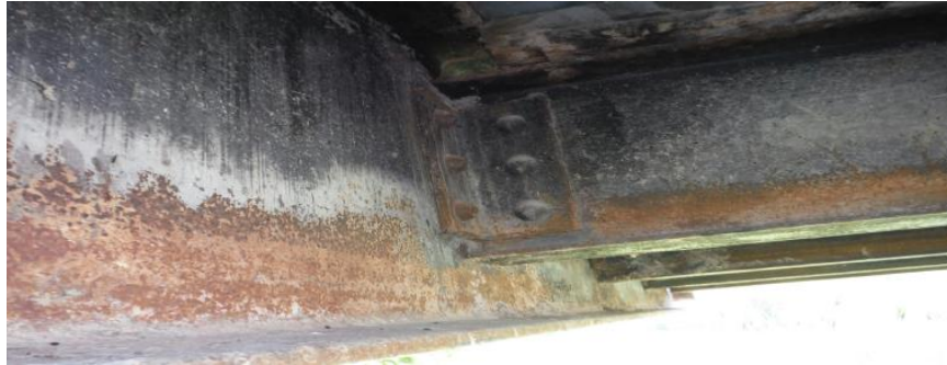
Figure 14: View of coating failure with corrosion on floorbeam, typical (courtesy of MDT)
