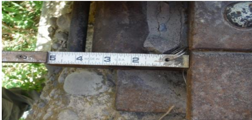
Figure 16: View of the south expansion bearing – roller nest extending 2 1/2" past masonry bearing plate (courtesy of MDT)
