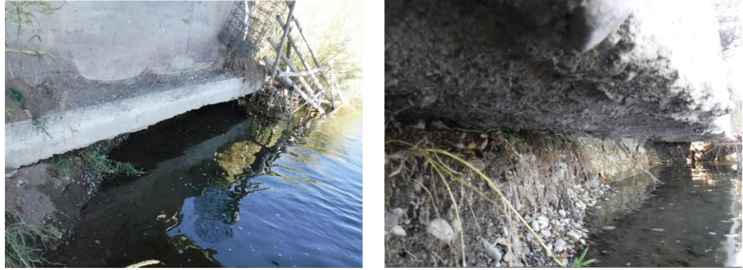
Figure 5: View of undermined Abutment 1 in 2019 (courtesy of MDT)
