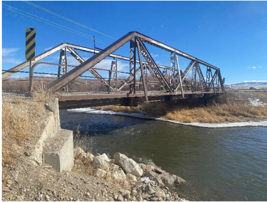
Figure 4: General view of steel Pony truss superstructure.
